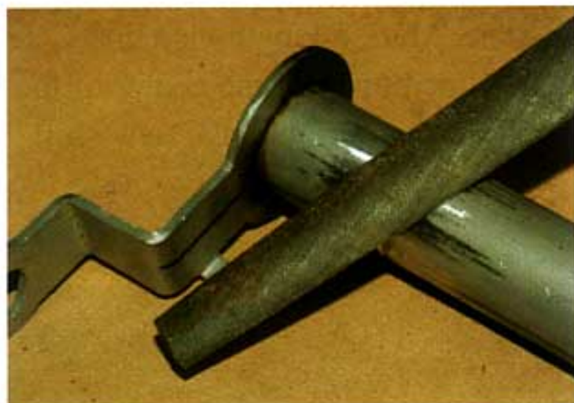
Photo #13: Use a flat file to dress up the lower part of the shift tube to make sure there is no welding slag.
